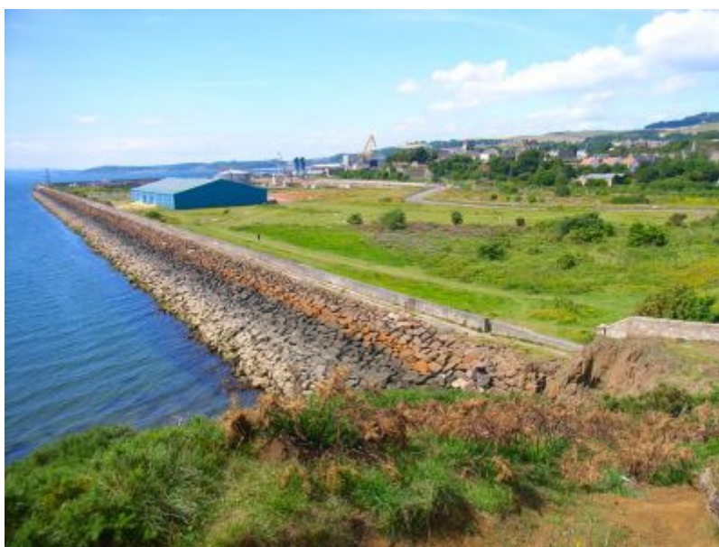
Above left - the Black Rocks viewed from the Lammerlaws at low tide, with the volcanic plug of the Bass Rock in the distance. Above right - close-up of the Black Rocks, with the Binn in the background. Below - breakwater, constructed with dolerite blocks from the Lammerlaws quarries.
